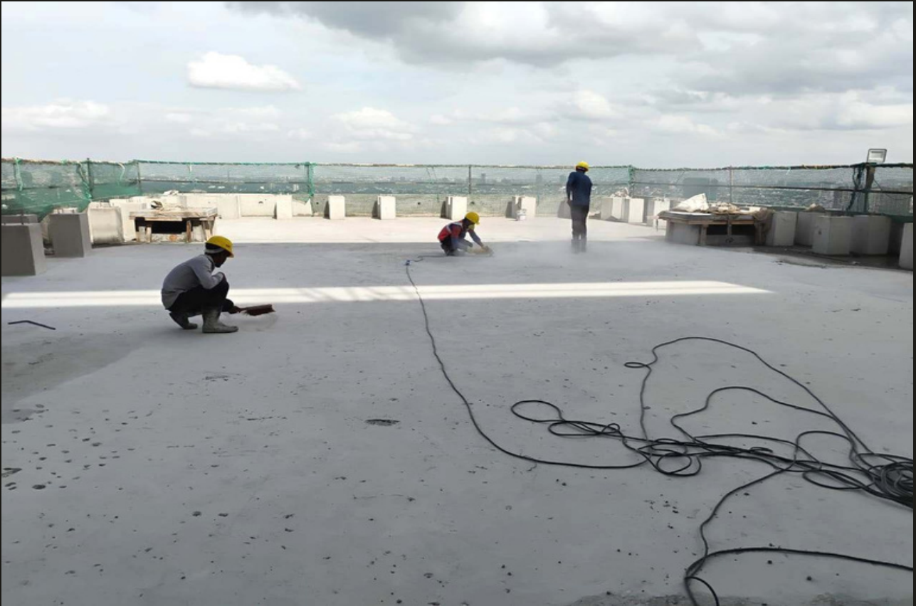
5. Tower-A terrace waterproofing grinding chipping work in progress
