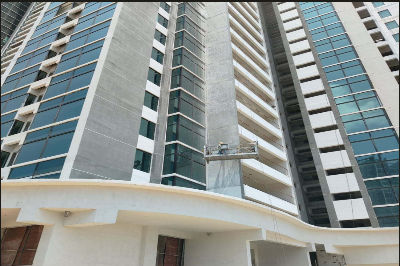
28. Tower B External painting work in progress
