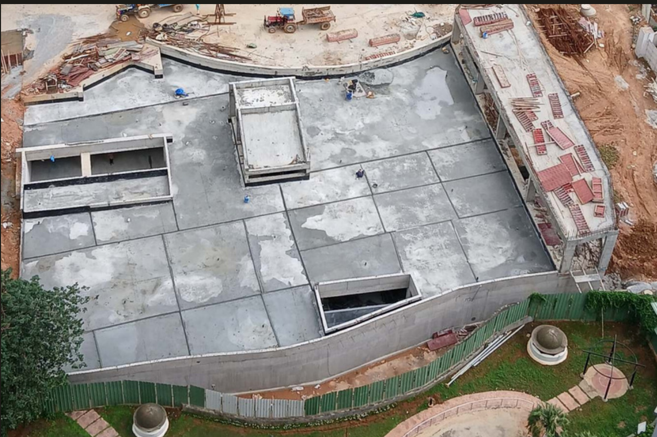
6. East side podium waterproofing protection screed concrete completed
