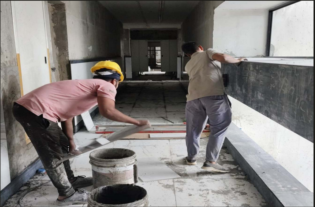
11. Tower A 31st Floor corridor dado tiling work in progress
