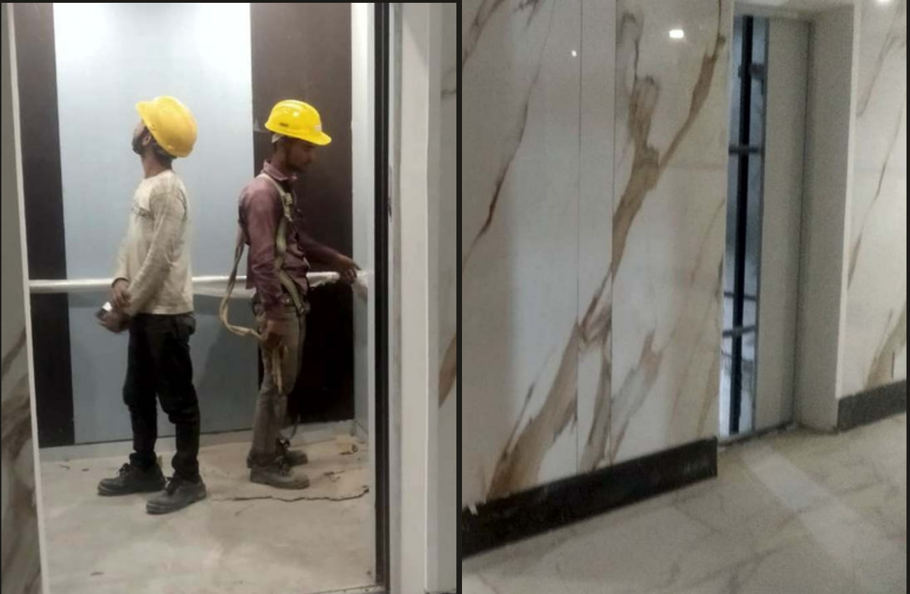
30. Tower B lift work in progress
