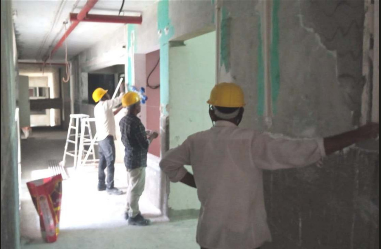
15. Tower B 12th Floor corridor gypsum bull mark work in progress
