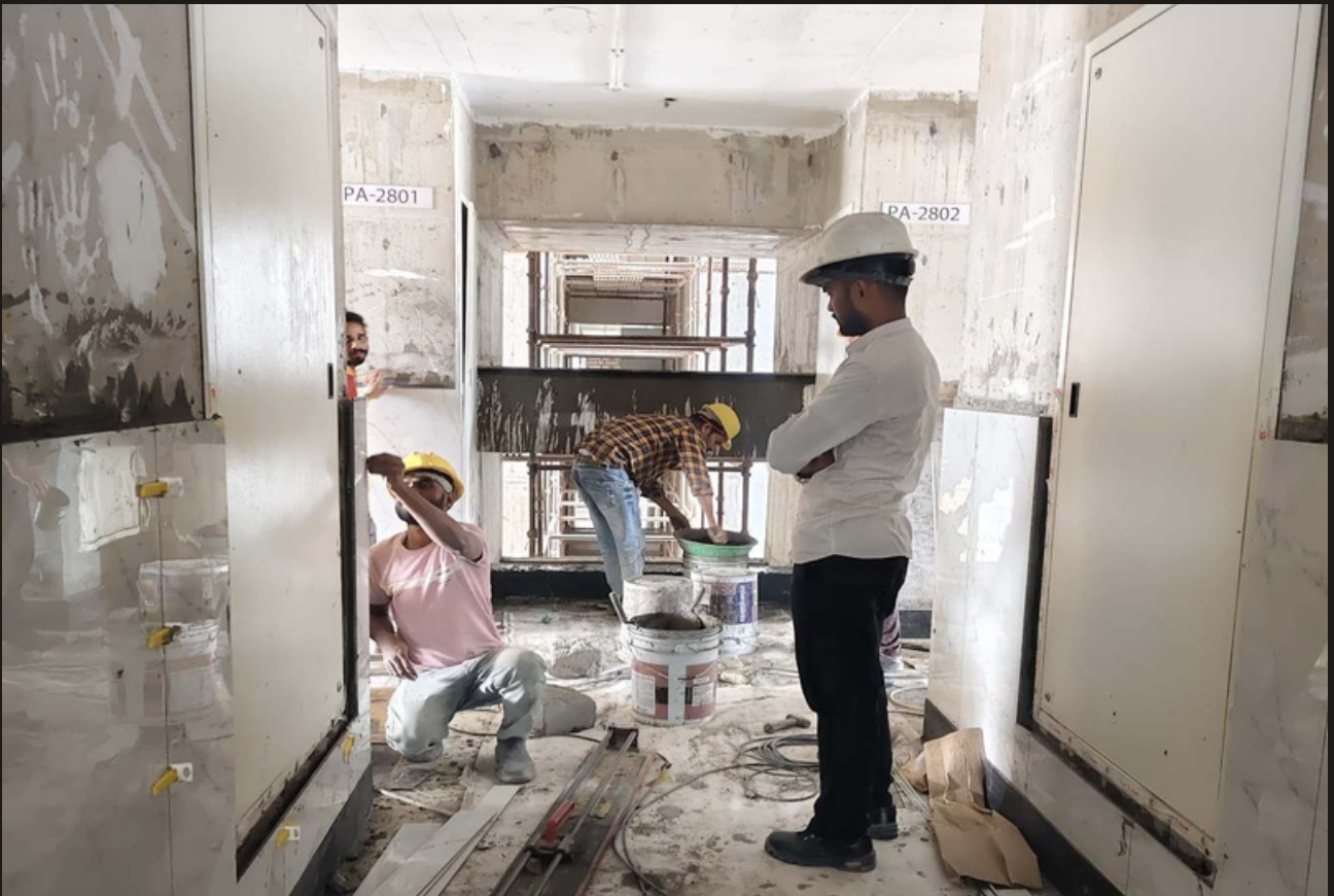
12. Tower A 28th Floor corridor dado tiling work in progress
