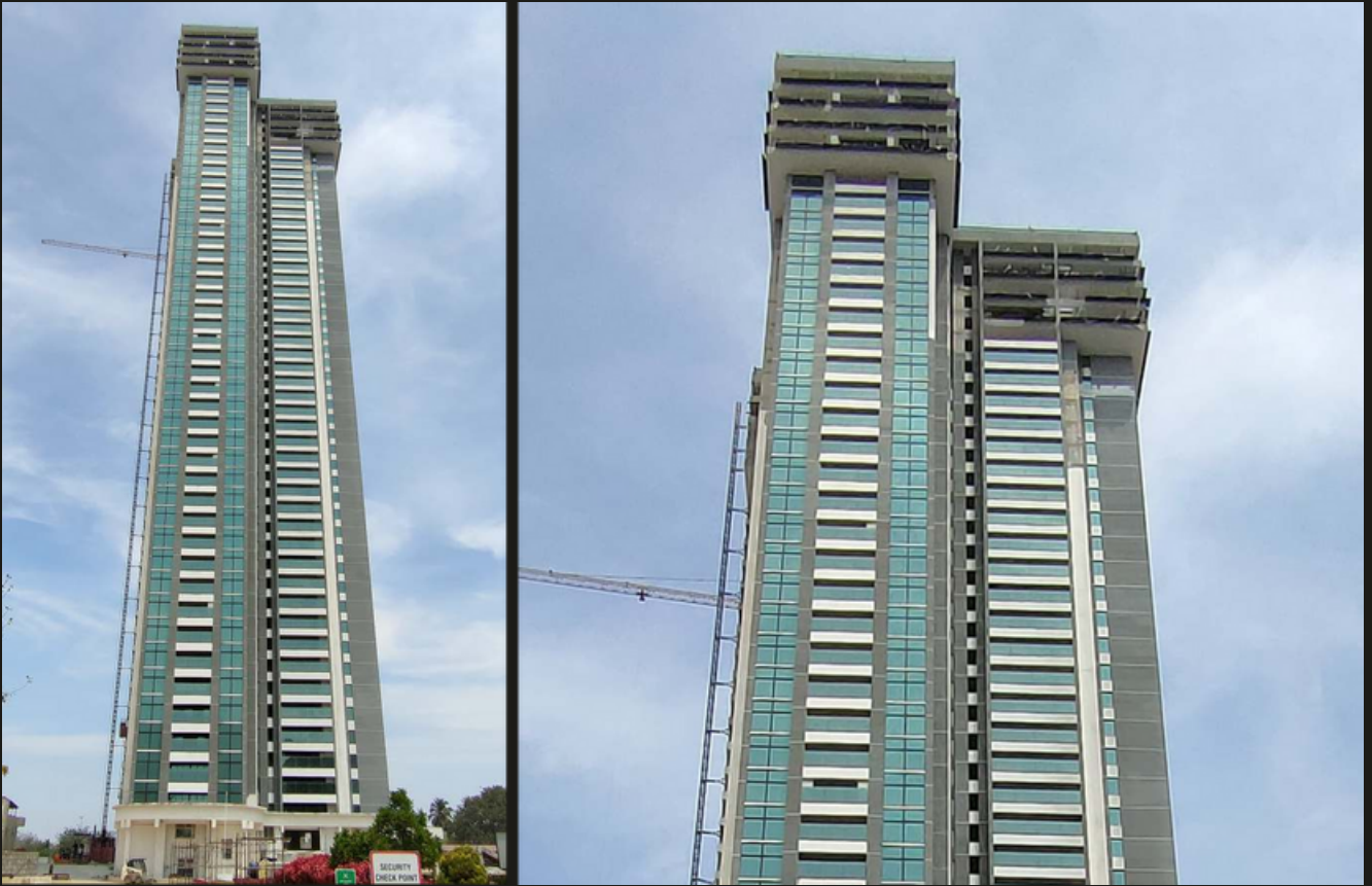
31. Tower A South face window glass & Balcony railing glass fixing complete
