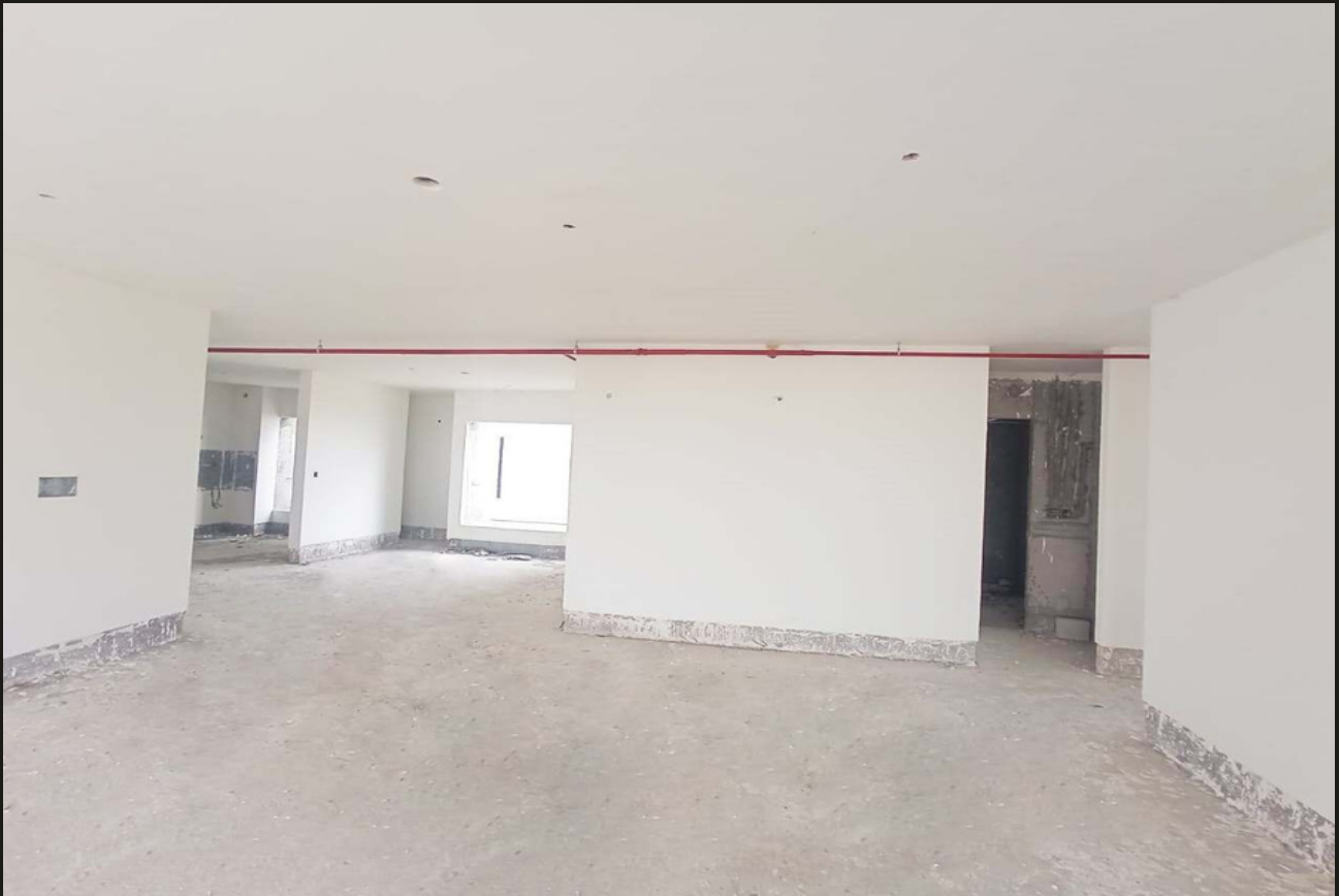
25. Tower A 28th Floor fire sprinkler work in progress
