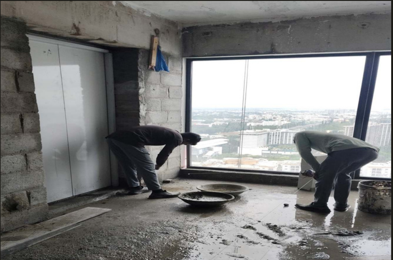
9. Tower A 35th Floor lift lobby bull marking for plaster work in progress
