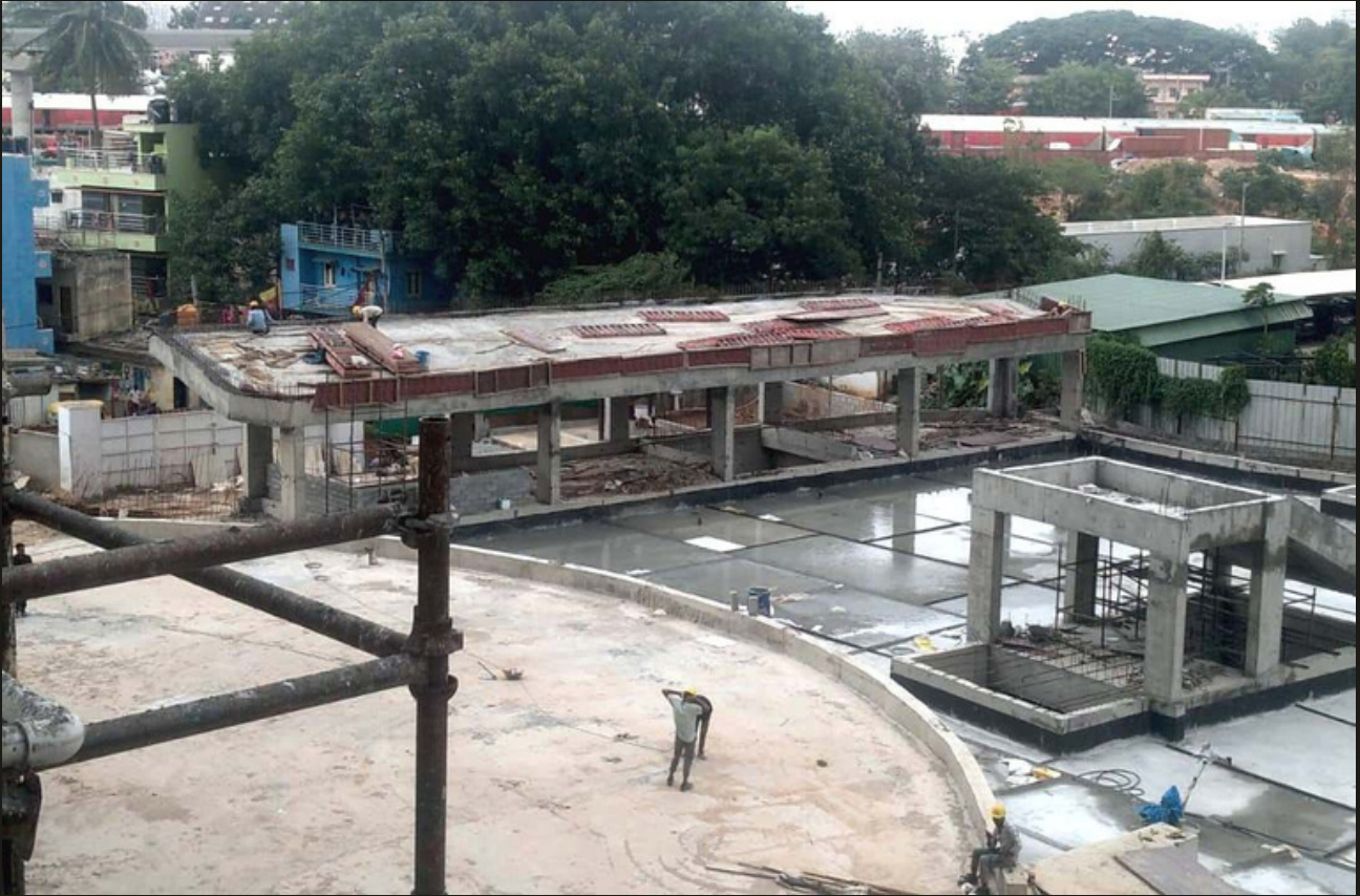
33. Fan room parapet wall work in progress
