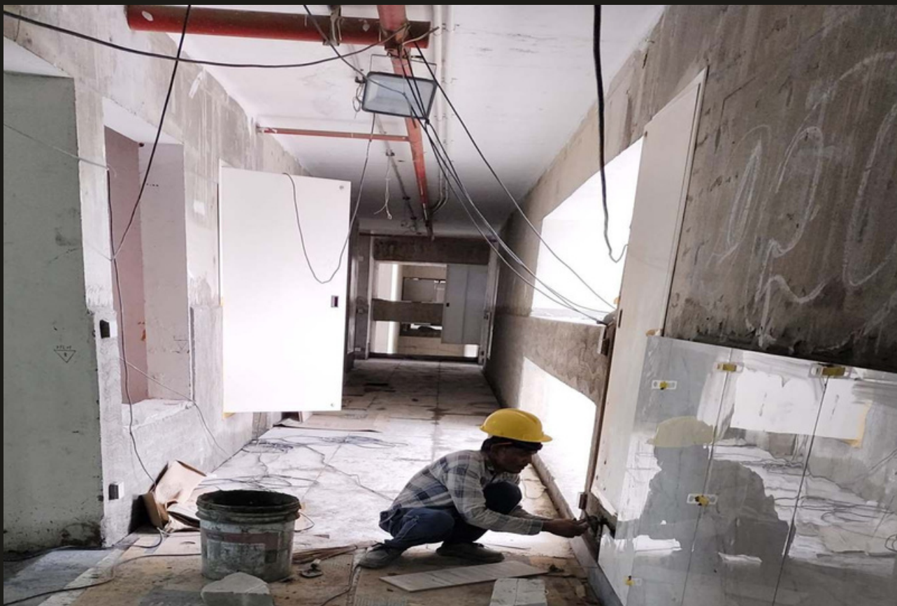
17. Tower A 20th Floor corridor tile work in progress
