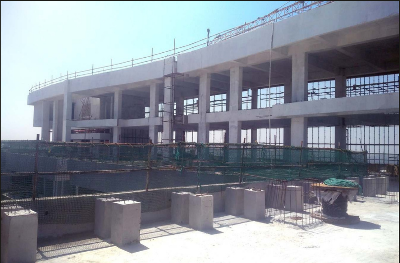
3. 50th floor Tower A Above Terrace painting work in progress
