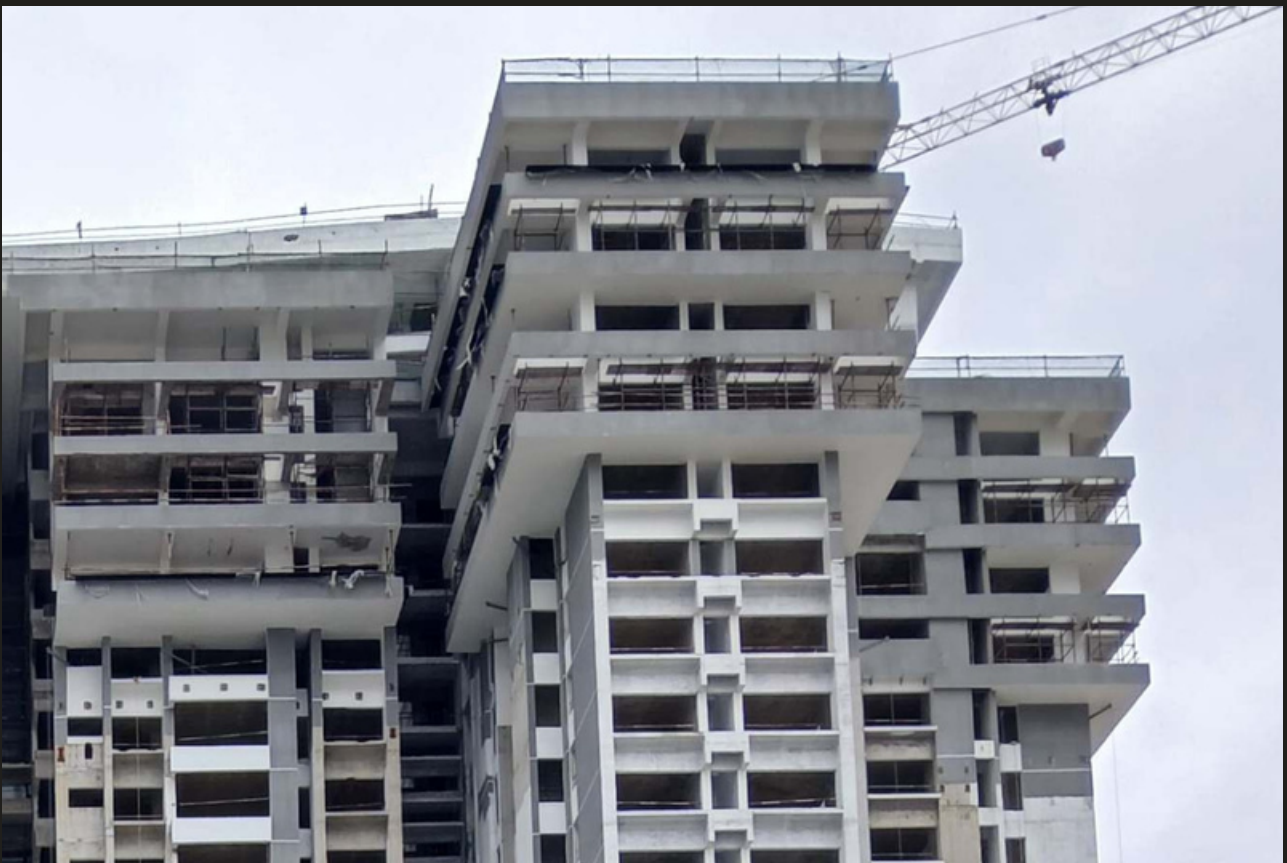
2. 45th floor Tower-B above external texture painting work complete
