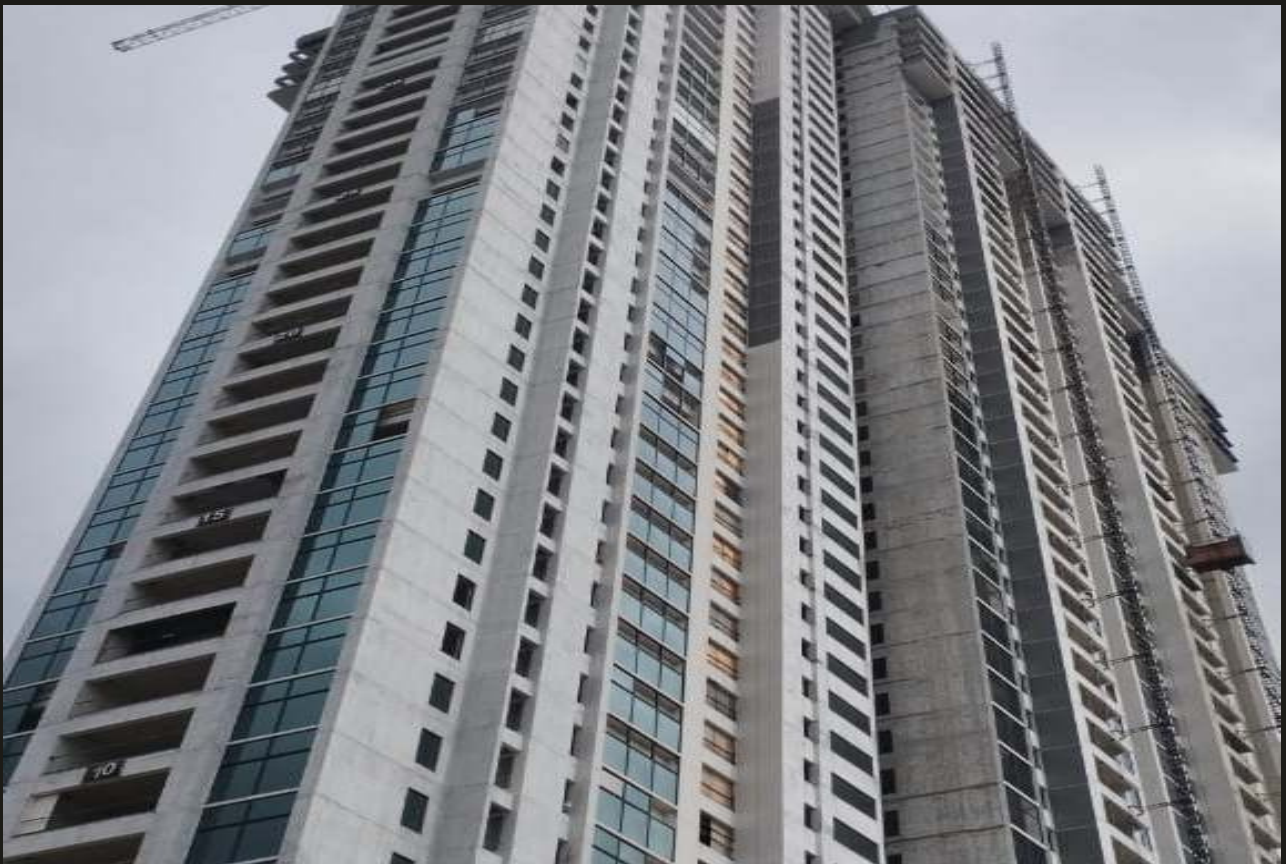
32. 29th Floor Tower B window glass fixing work in progress
