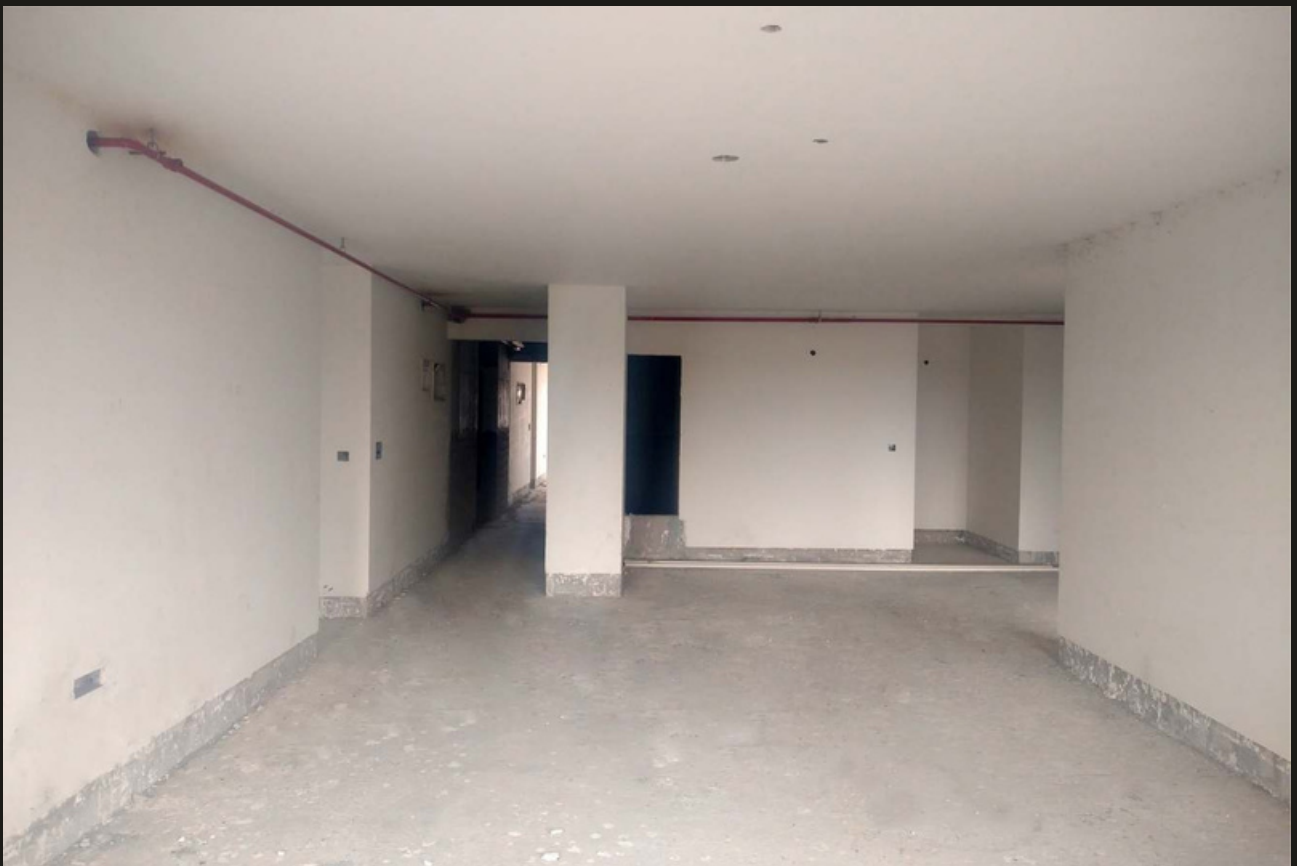
26. Tower B 28th Floor fire sprinkler work in progress
