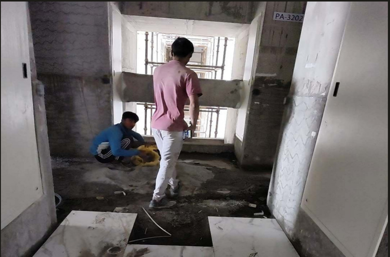
20. Tower A 32nd Floor corridor tile work in progress
