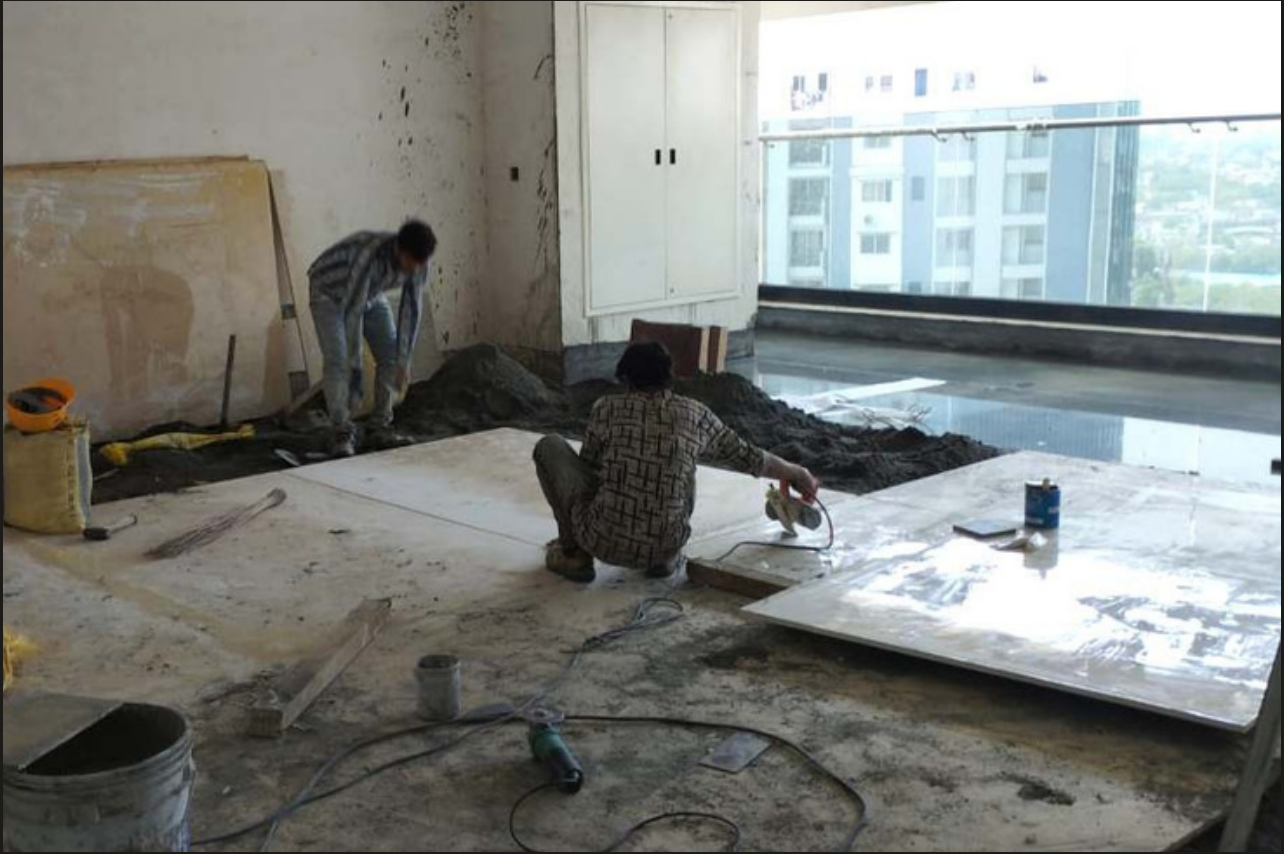
21. Tower A 18th Floor Marble flooring work in progress
