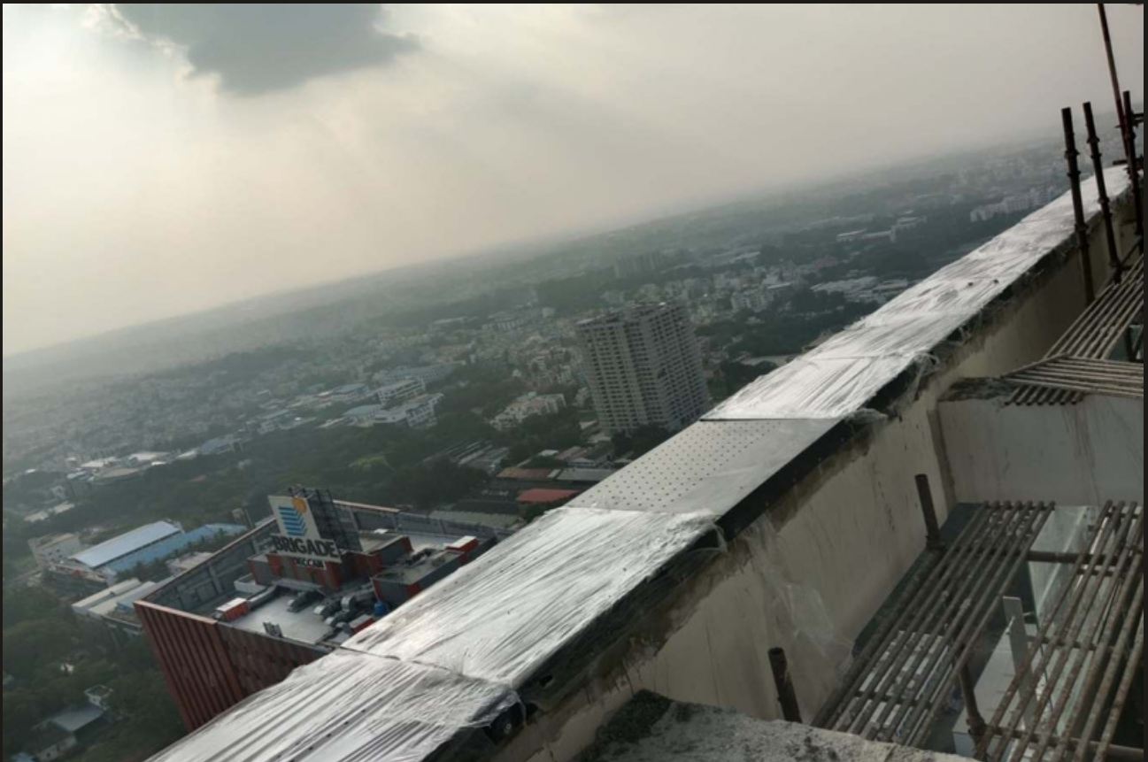
38. 47th floor Tower A fin fixing in progress
