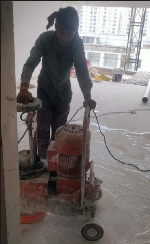
22. Tower A 7th floor marble polishing work in progress
