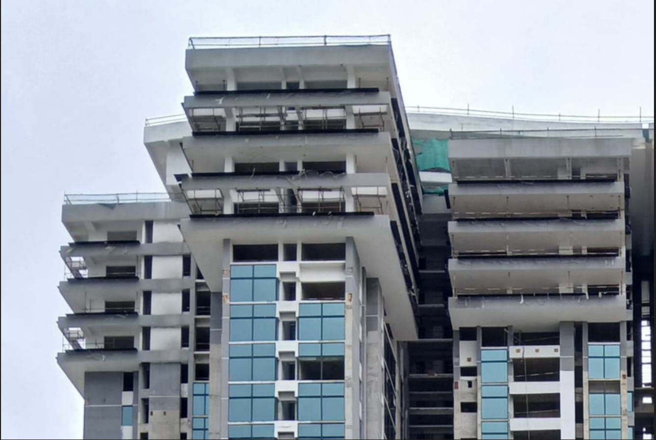
1. 45th floor Tower-A above external texture painting work complete
