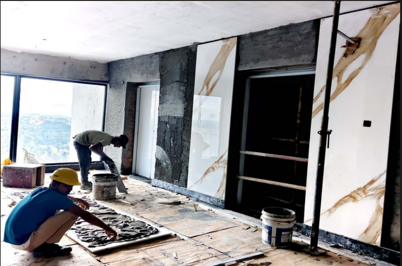
27. 6th floor Tower A Lift lobby wall cladding work in progress
