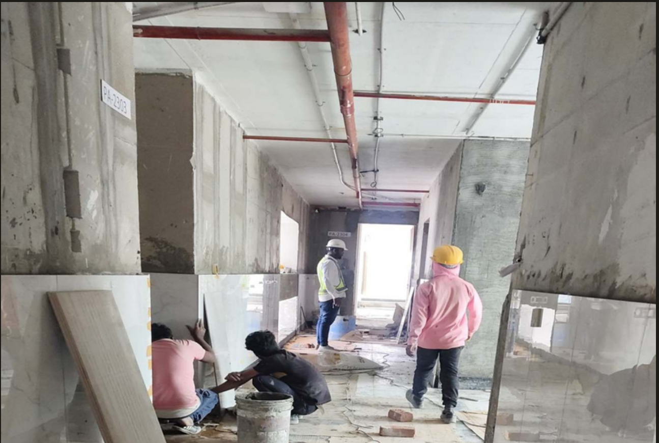
10. Tower A 23rd Floor corridor dado tiling work in progress
