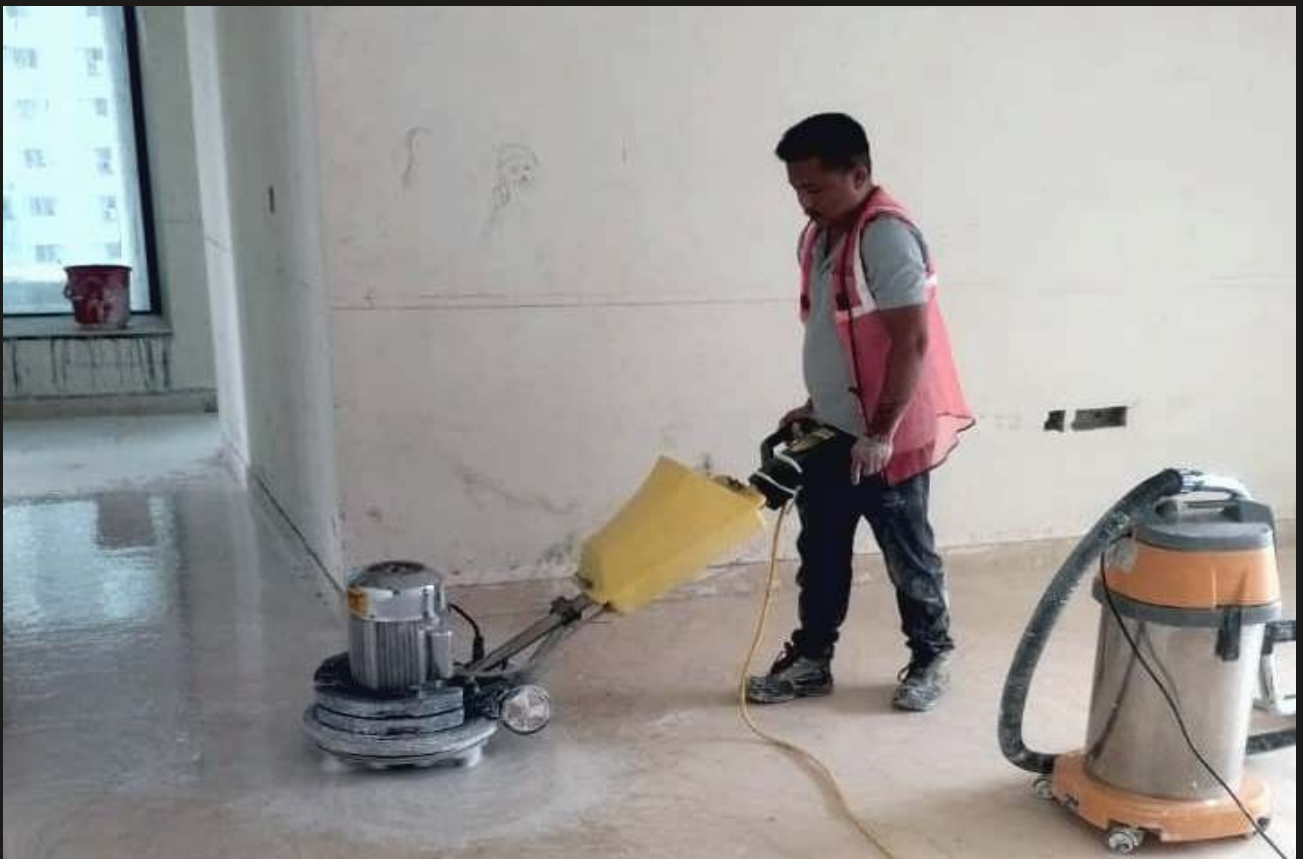
16. Tower A 903 marble polishing work in progress
