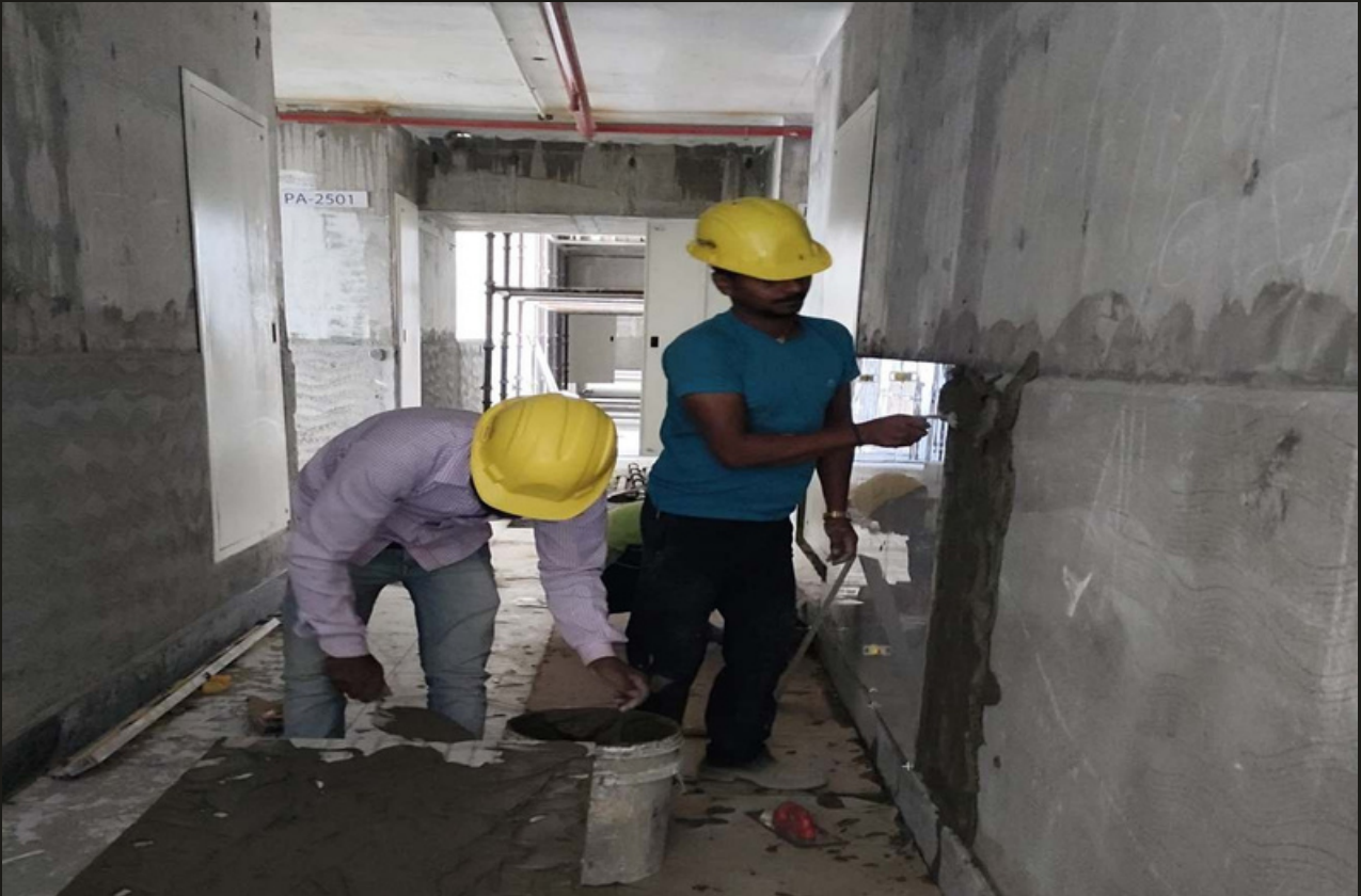
13. Tower A 25th Floor corridor dado tiling work in progress
