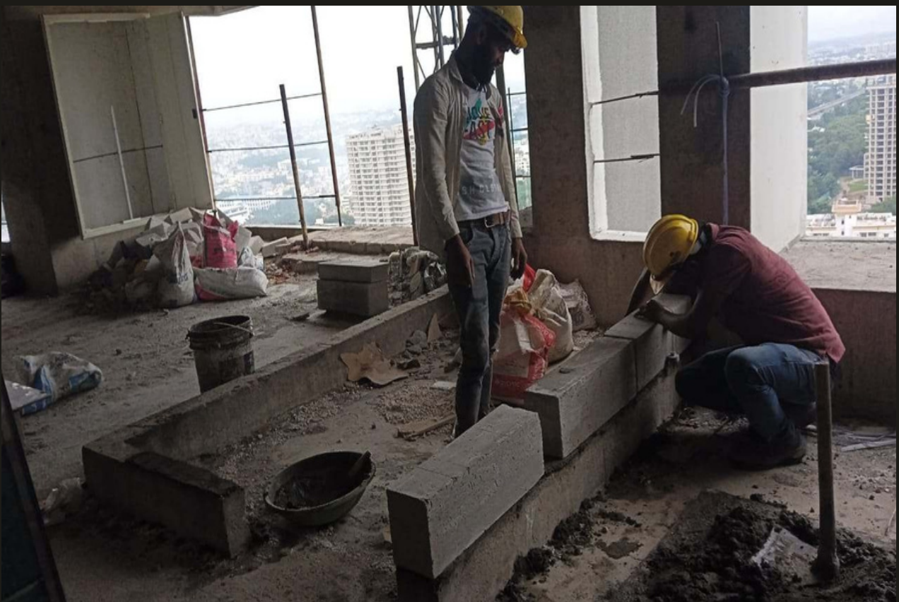
24. Tower B 3101 base coarse marking in progress
