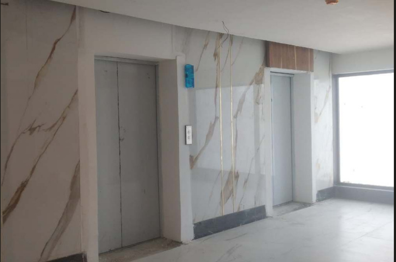
29. Tower A 2 lift operational
