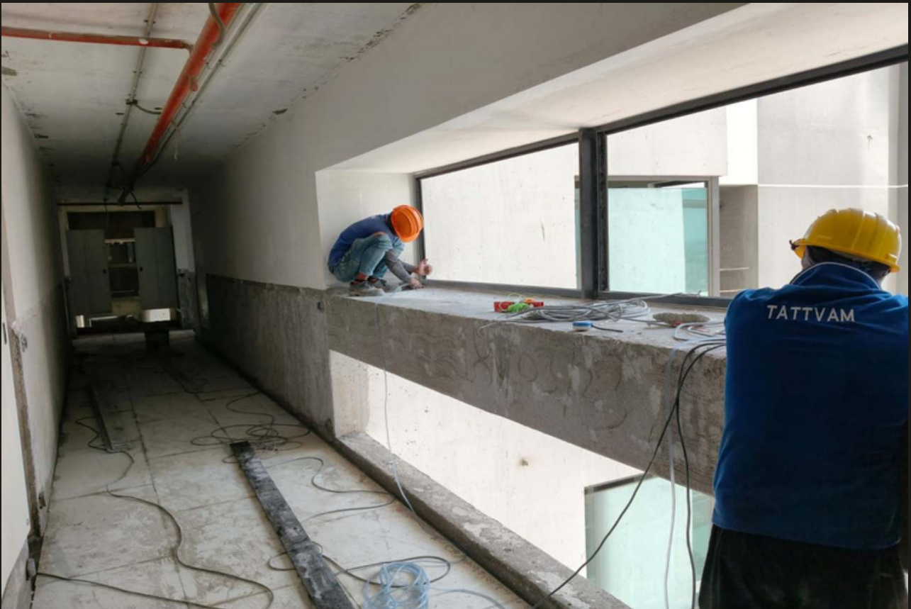
23. Tower A corridor window frame fixing in progress
