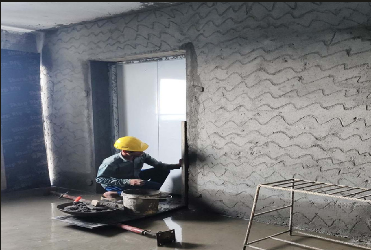
18. Tower A 43rd Floor lift lobby brick work and plaster work in progress
