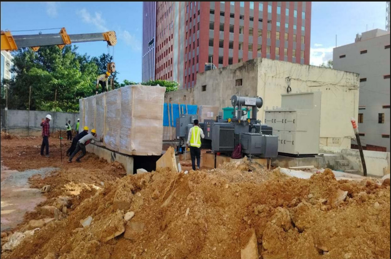
8. Power panel delivered to site
