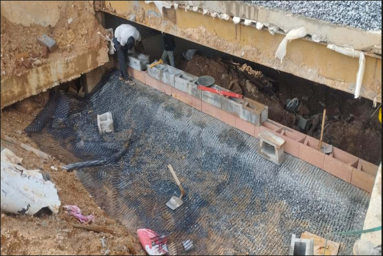
7. West side Retaining wall work in progress
