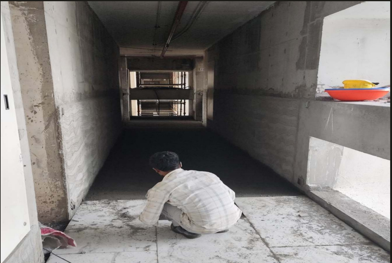
14. Tower A 26th Floor corridor floor tile work in progress
