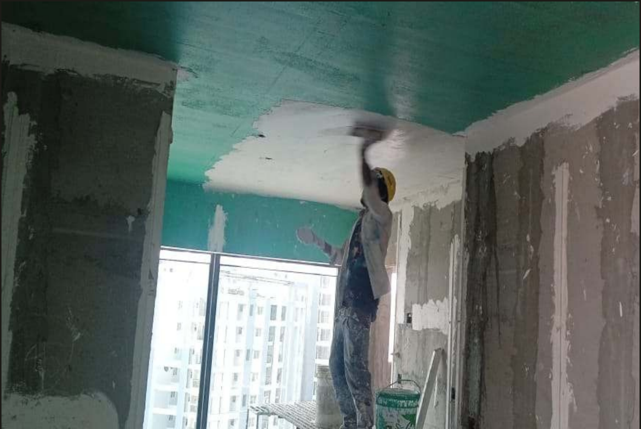
19. Tower B 1902 ceiling gypsum plastering work in progress
