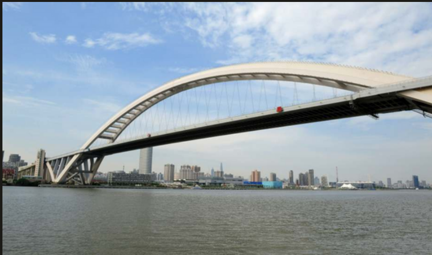
Shanghai Lupu Bridge
